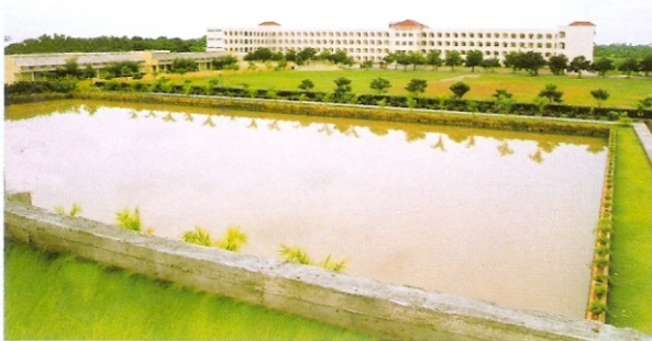
A Panoramic view of buildings with rainwater plant
